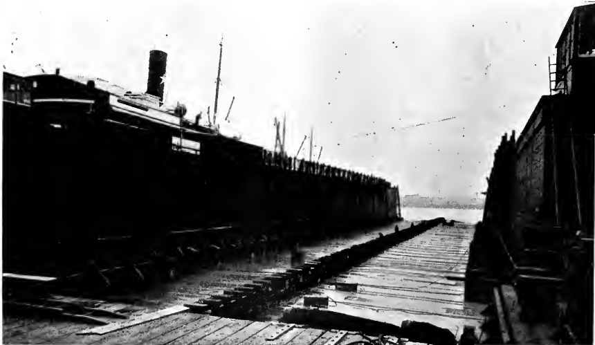
The latest addition to the Union Iron Works dry dock equipment, a large floating dock just completed.
